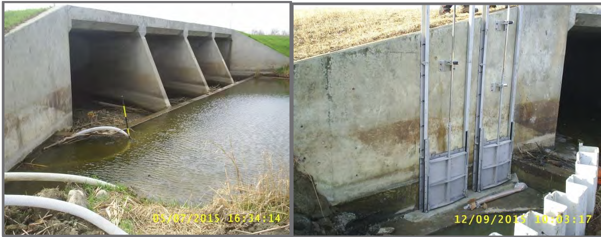
Figure 5: Diversion Structure and Base Flow Gate System
