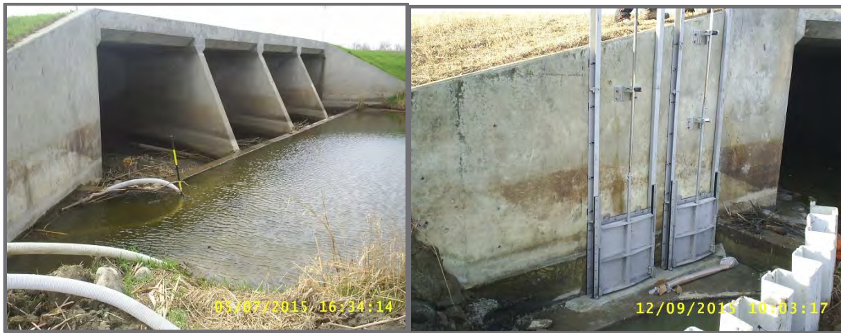
Figure 5: Diversion Structure and Base Flow Gate System
