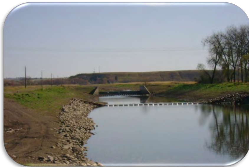
Figure 6: Drop Structures in the Diversion Channel – Looking East
