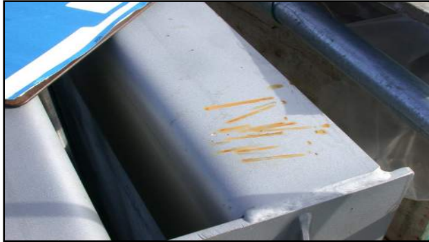
Contamination caused by grinding nearby
