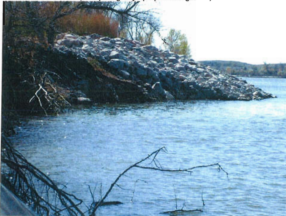
View South 2830 Langer Way Shoreline October 2, 2011 (Whispering Bay riprap in background)
