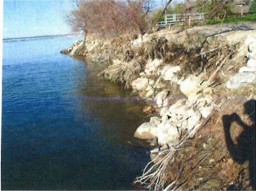
View North 2830 Langer Way Shoreline October 1, 2011
