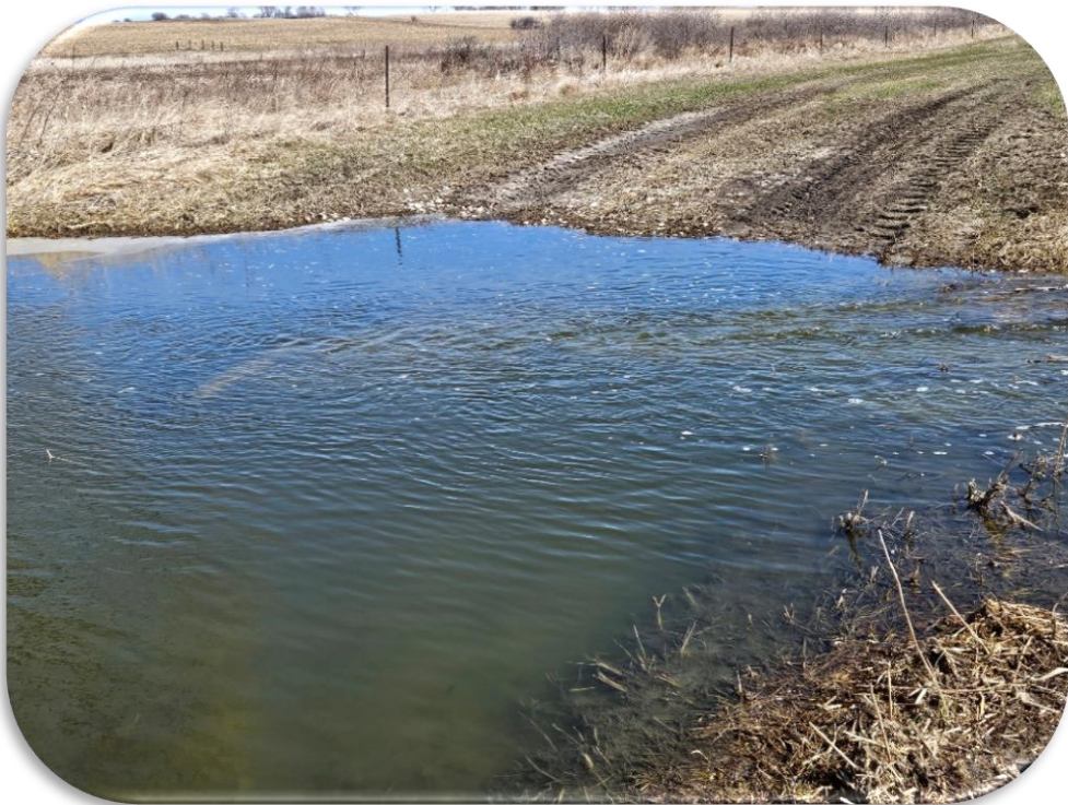
Location of township roadway easement and Texas crossing shallow gravel base Some cleaning appears to have been done in this area, mostly on the north side.
